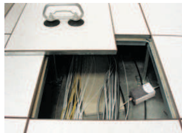
Filtering Ground in Subfloor
